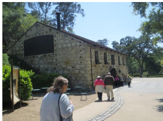
Heading toward original, restored building of Buena Vista Winery
